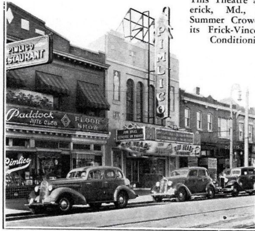
The 1200-seat Pimlico and the 650-seat Irvington Theatres, both in Baltimore, alike use Vincent Air Conditioning to Advantage.
